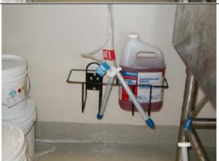
17. Insert the 1 gallon bottle of product in the rack and insert the product supply tube assembly.
