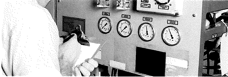
Buildings #1, 2, 4 & 5 Test & Balance
