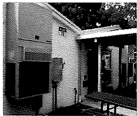
Electrical lighting improvements in building 78.
