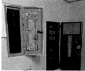
Replacements of old electrical panels in building 1.
