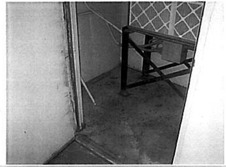
See required corrective action page Line # 34
