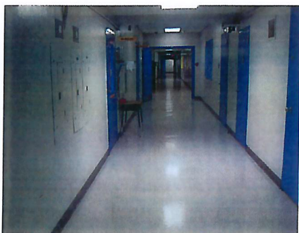
VCT flooring in hallways glossy
