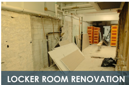
RELOCATION OF DRAIN LINE
